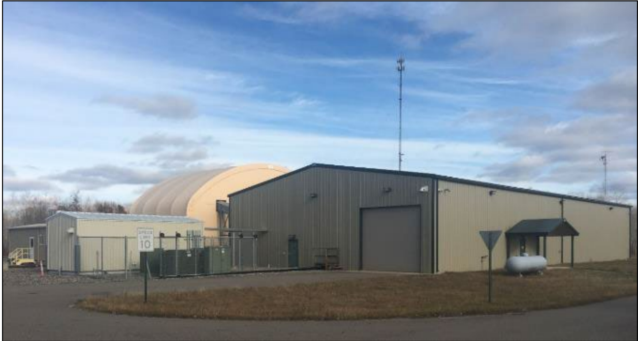
Figure 18-2 Ground view of the primary plant structures
