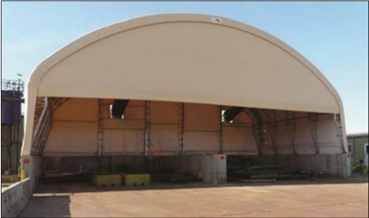
Figure 18-8 Material storage facility
