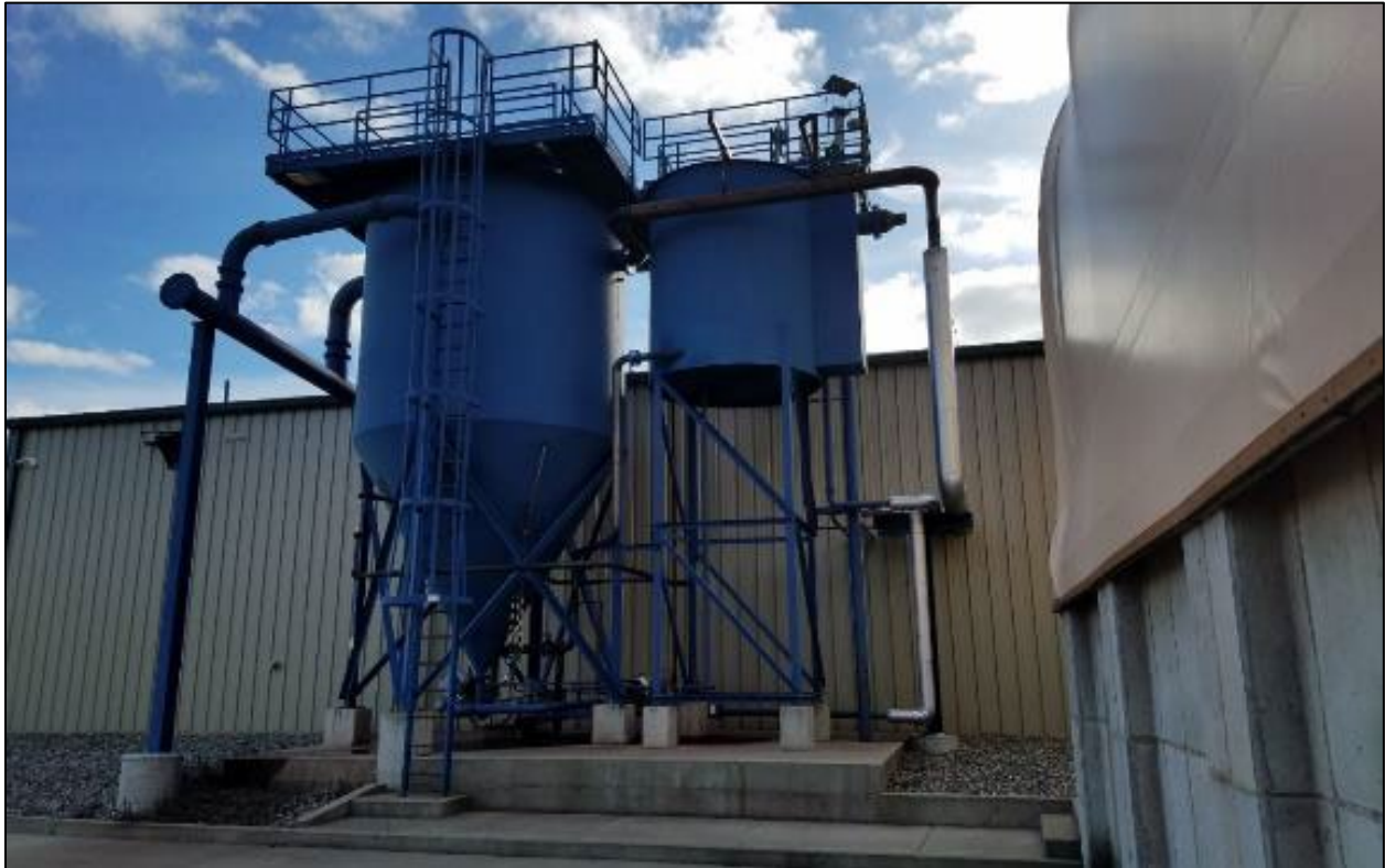
Figure 18-7 Clarifier tank
